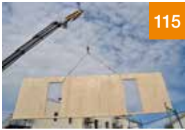
Transformation through a production system
